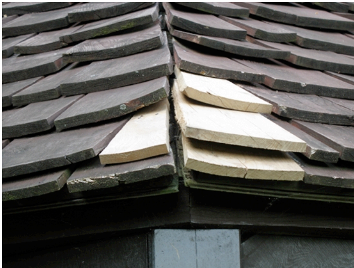
Repaired Shingles (Detail) - Hugh & Chris.
